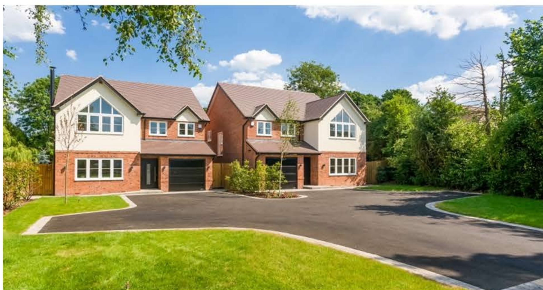
The Development Will Incorporate Green Infrastructure [Bio-Diversity Net Gain] - Refer to Drawing PL-16-Proposed Planting + BNG Plan + Cotswold Wildlife Survey Documents. The Proposed Scheme Will Incorporate New Native Hedgerows + Trees.
