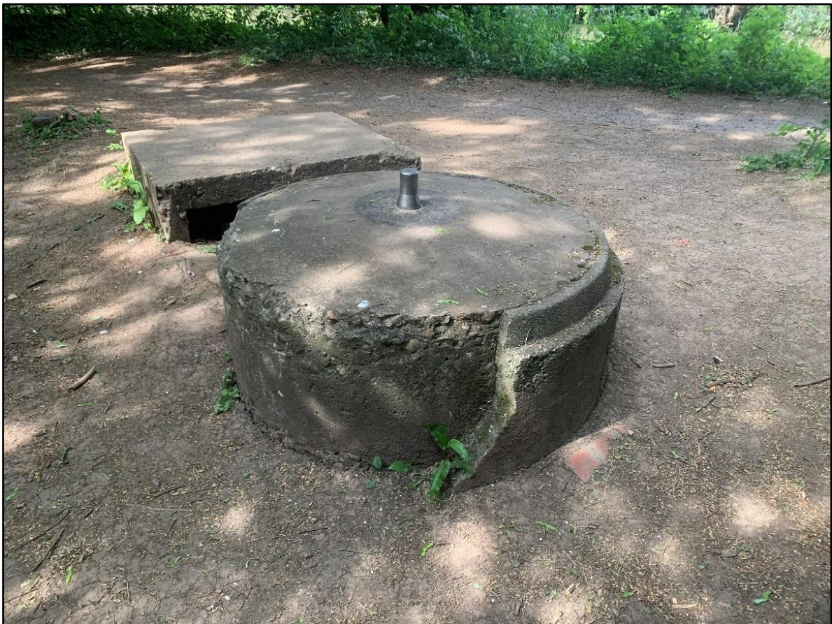
Figure 4: Spigot Mortar with ammunition locker at Oxford Canal, Shilton Lane (looking north-west)
