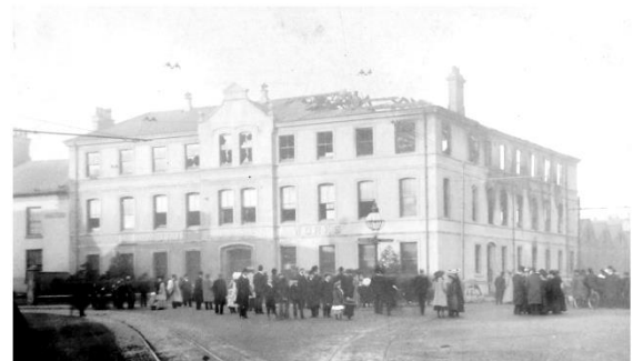
Figure 3. Image from 1906 following the fire at the Humber Motor Works, showing building pre-ground floor extension and rear section loss.
