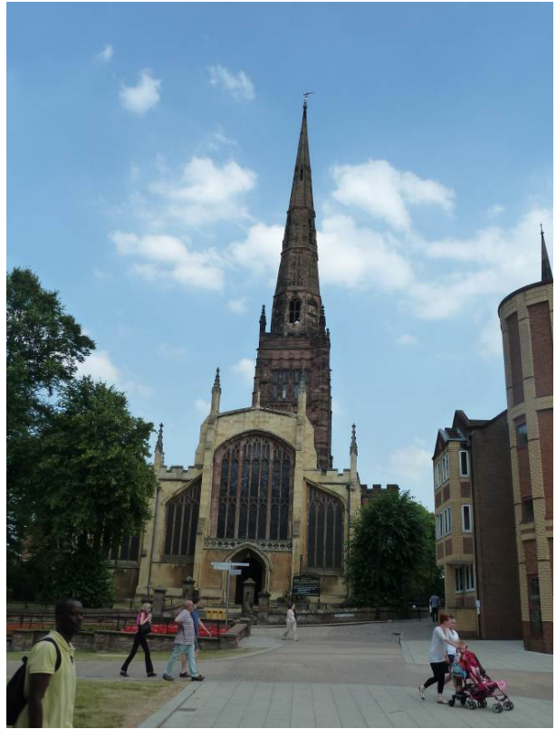
Holy Trinity Church viewed from Trinity Lane area
