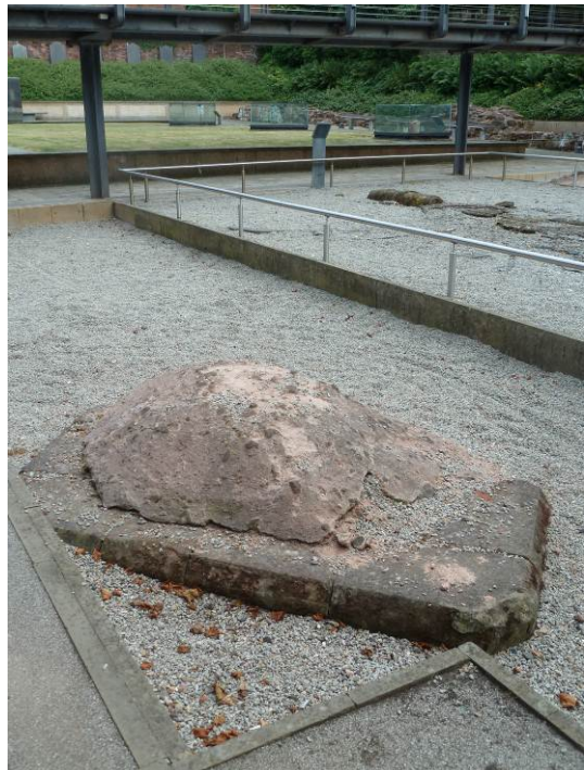
Damage to archaeological remains in Priory Gardens
