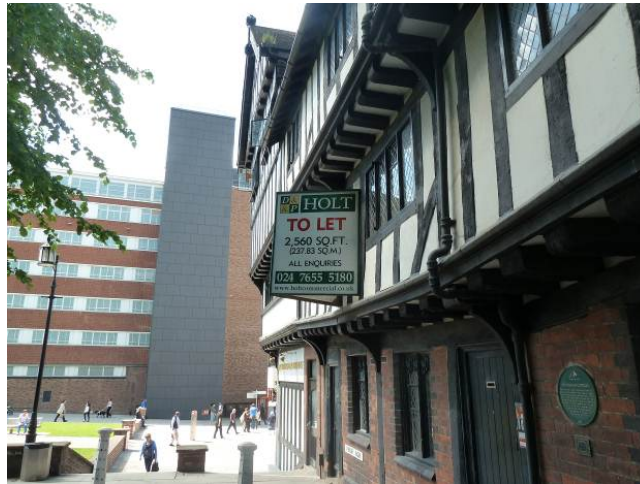
Unnecessarily large advertising boards attached to listed buildings
