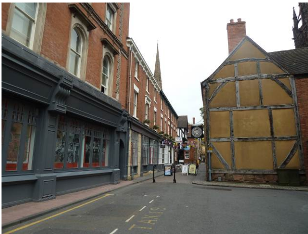
Nos. 1-6 Hay Lane, 19 th century brick buildings and the timber-framed gable end of no.10a
