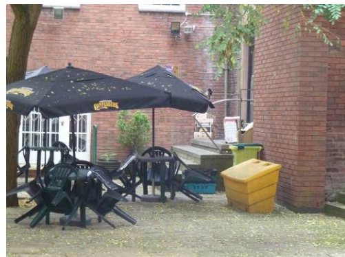
Rubbish left outside buildings in Castle Yard
