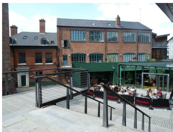
New Buildings, former ribbon factory
