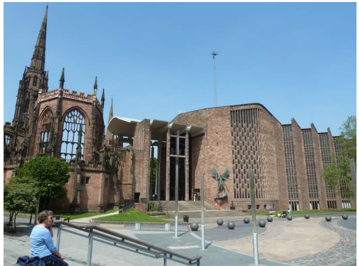
View of the old and new Cathedrals from University Square
