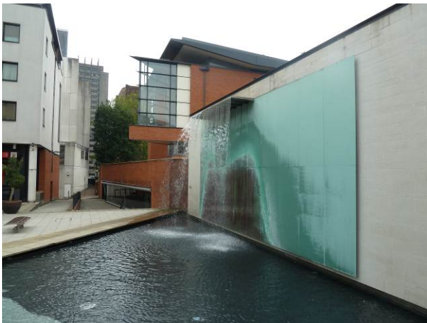
Waterwindow installation from Priory Place (above) and from the Cloister Garden (right)
