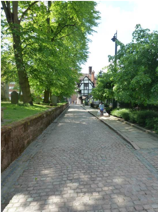
Cobbled street surface on Priory Row
