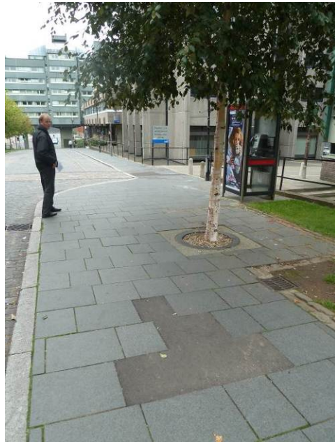
Repairs to paving slabs on Priory Street
