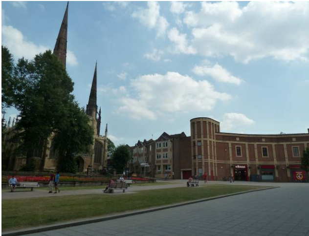
Cathedral Lanes shopping centre which impacts negatively on the view of the conservation area
