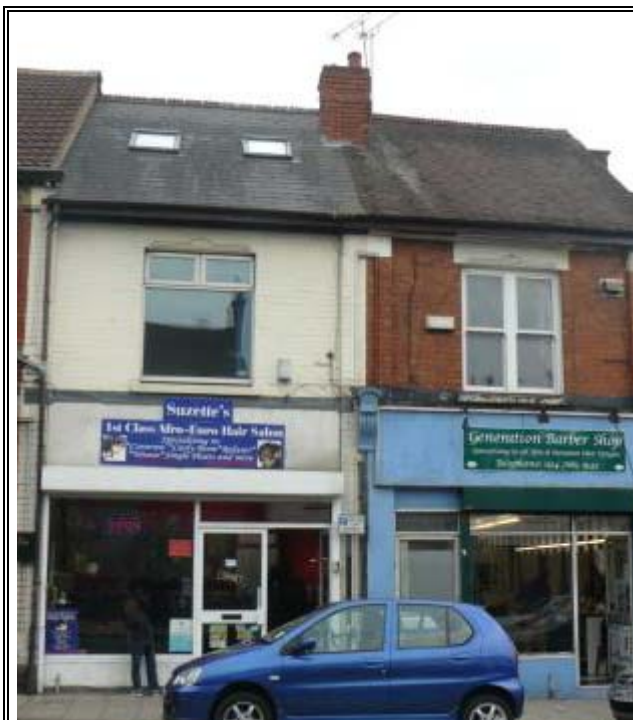
Rooflights and Wiring
