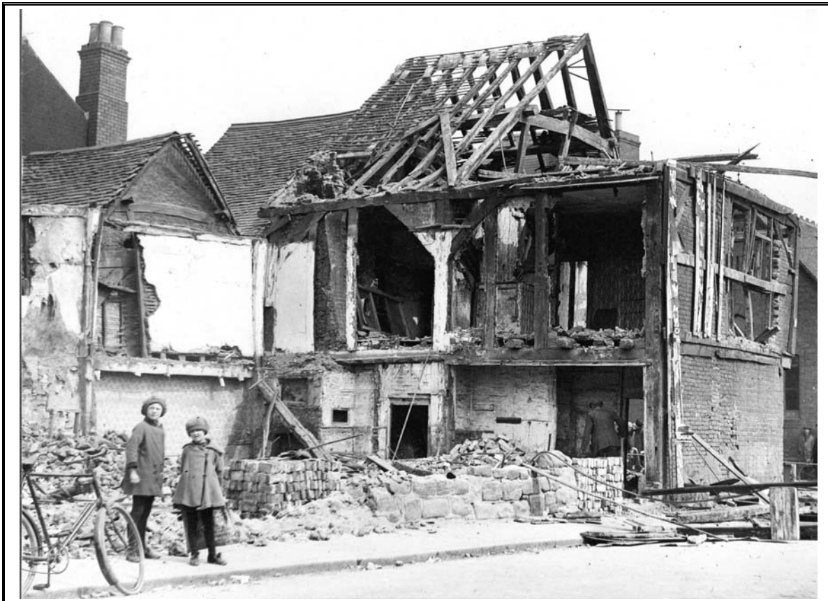
Demolition of Nos. 26 and 27 Far Gosford Street
