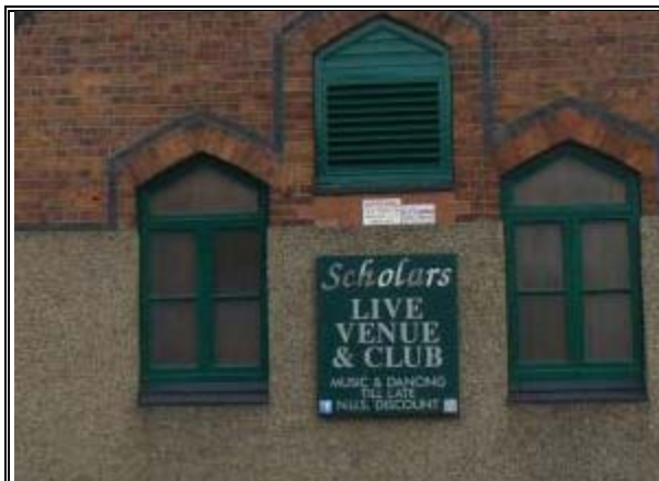
Windows to the former All Saints' School
