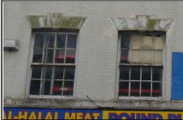
Sash Windows to Number 93
